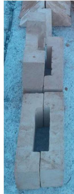
*Picture 7: Cut bricks for P channel port lintel.*
