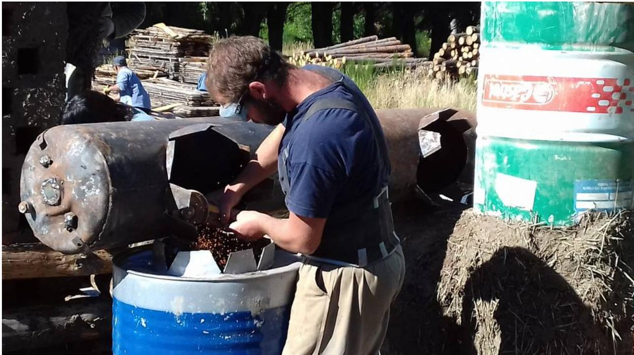
*Picture 19: Detail of the connection piece between the heat riser and the descent tower. Made of what's available in place (better materials than proposed in the plans). 2 discarded woodburning steel boilers.*
