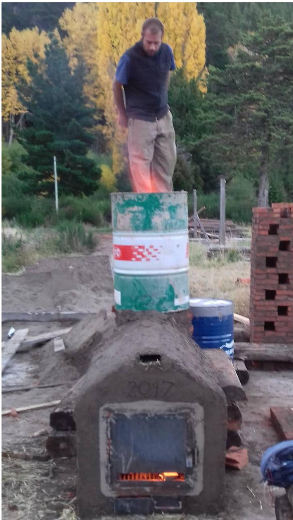
*Picture 9: Firebox coated and heat riser at planned height (1,80m; 7,5B). Ramiro facing down. On the right, one of the twin towers rising.*
